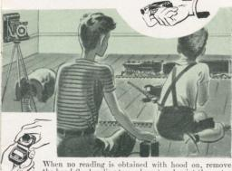
When no reading is obtained with hood on, remove the hood (by bending toward you) and point the meter at the camera, from the subject, and read light value indicated.
